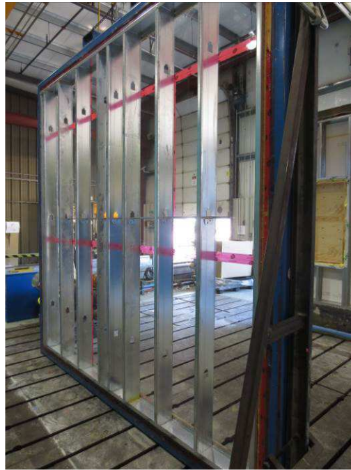
Figure B1 – Backup Wall Framing and Plexiglas Installation
