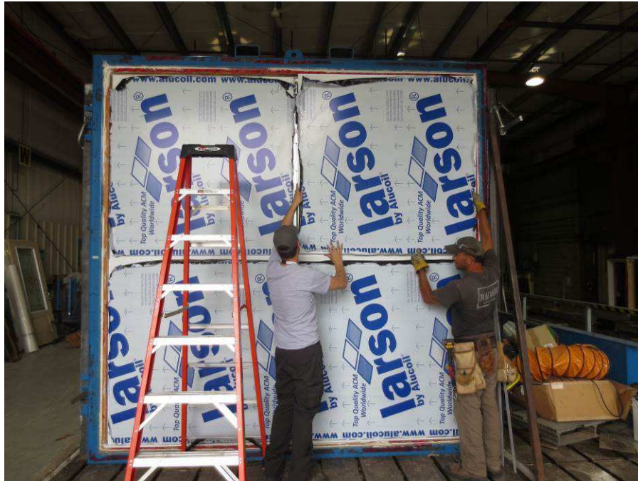
Figure B3 – Upper Panel Installation
