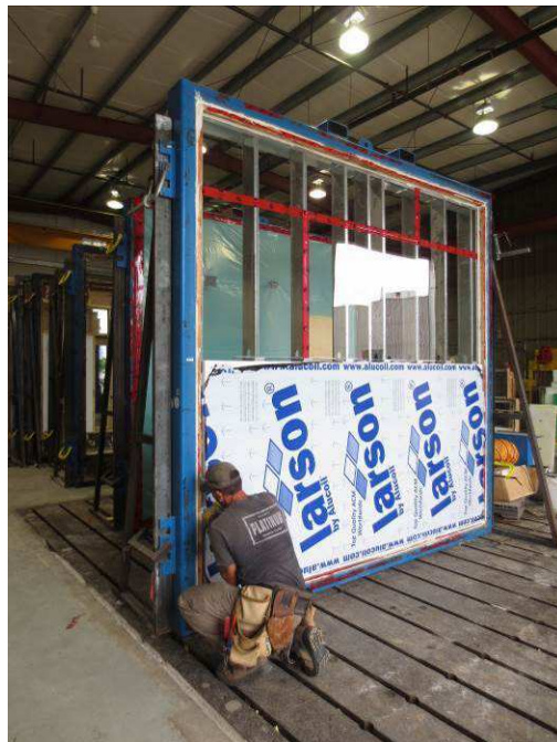
Figure B2 – Lower Panel Installation
